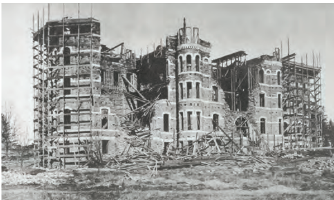
Collapse of Saint Joseph Hall, November 1900.
